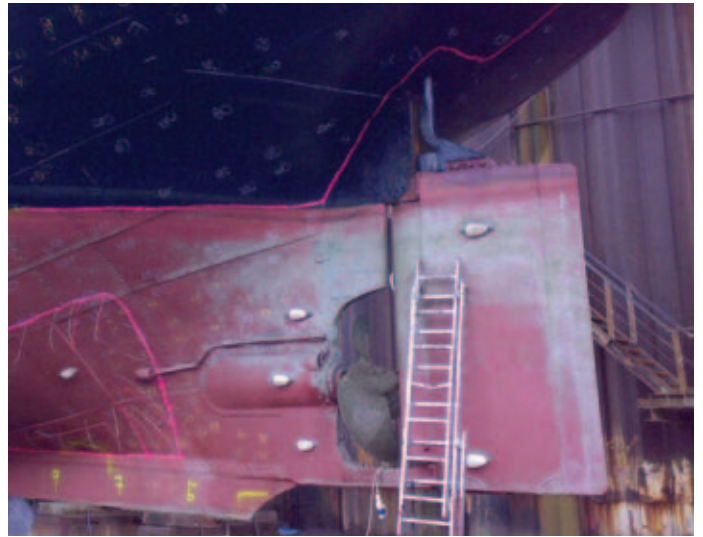
FIG.2: Some 3,000 points and defined lines were scanned during the hull survey
